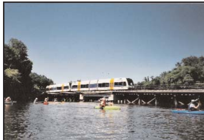
RiverLINE across Crosswicks Creek
