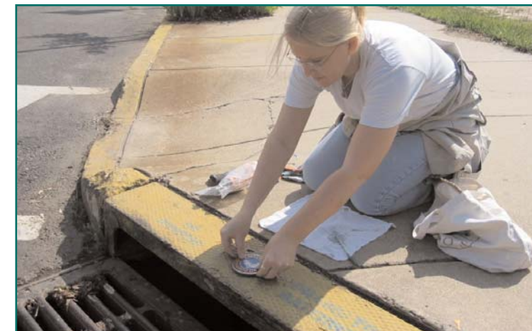
Volunteers installed 60 storm drain markers
